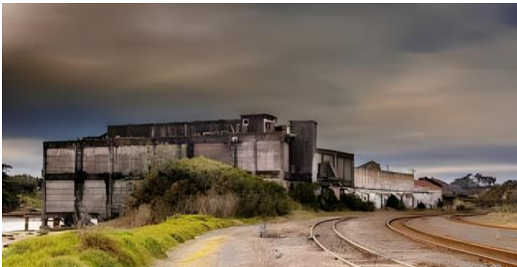
Patea Freezing Works - abandoned
