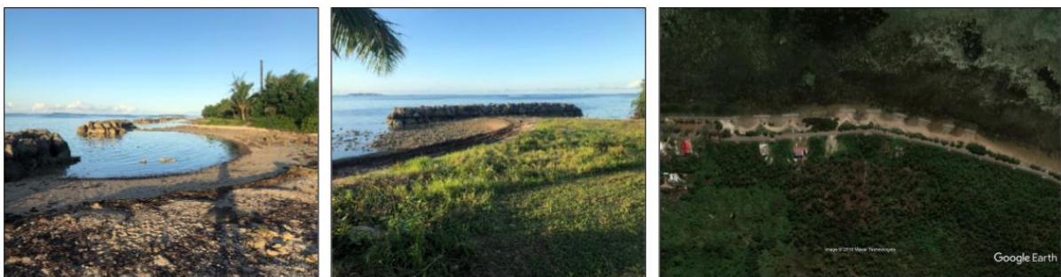
Figure 3: The detached breakwaters at Manuka, which have been extremely effective at widening the beach to provide a buffer zone and stop over-topping onto the road. There is now 10 – 30 metre of buffer zone and a series of crescent shaped beaches.
