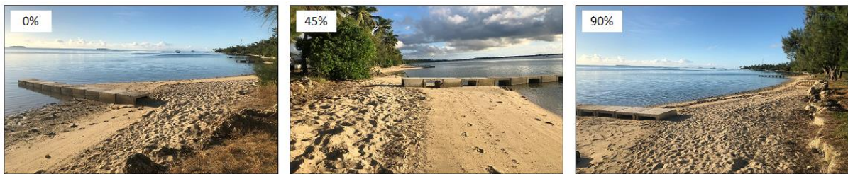
Figure 2: The groynes spaced along the beach with varying degrees of permeability (i.e. impermeable, 45% permeable, and 90% permeable).
